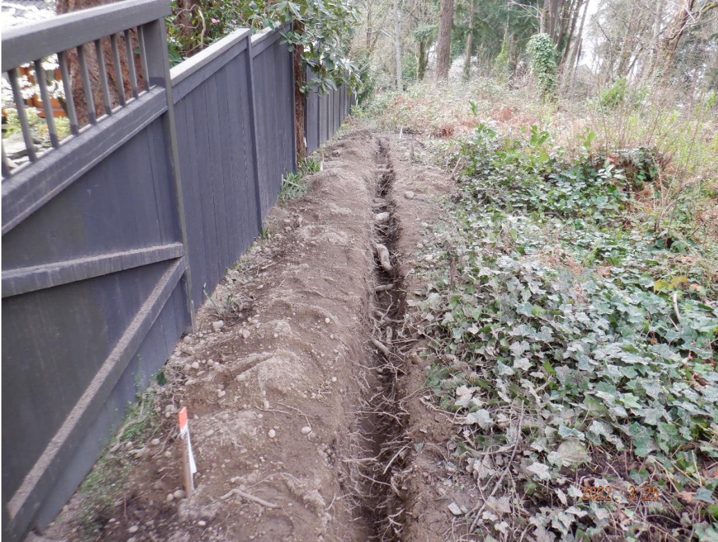
Trench air-excavated at excavation extent along east property line
